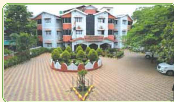
Sadar Dak Bungalow - the existing building of the Jalpaiguri Circuit Bench
