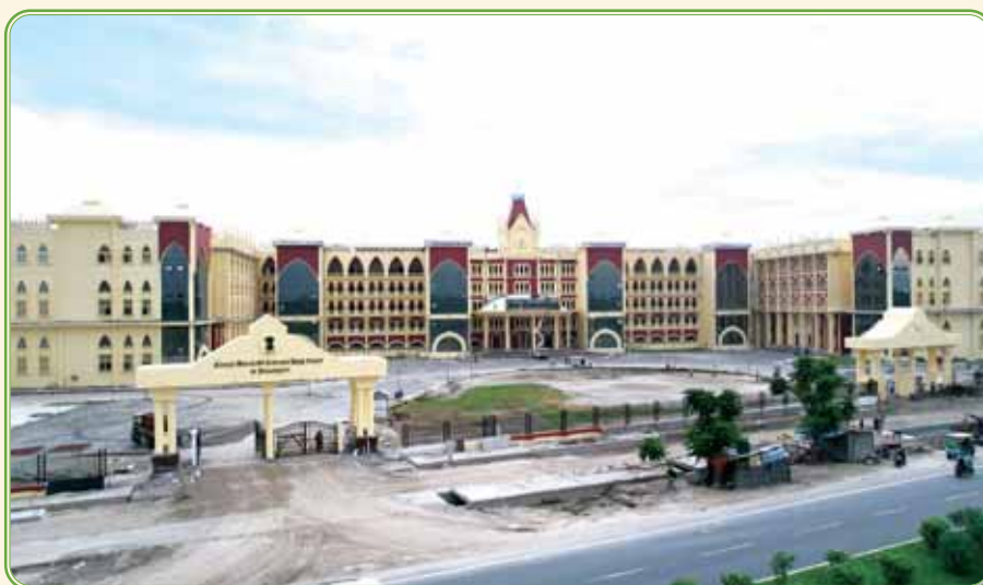
Panoramic view of the new building, beautifully designed in resonance with the iconic neo-Gothic architecture of the High Court at Calcutta
